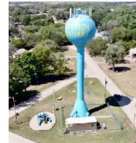
New Nickerson Water Tower
