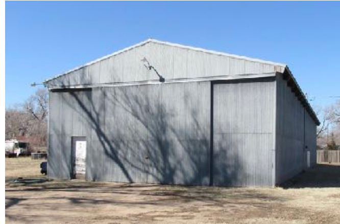
Nickerson Park Shop
