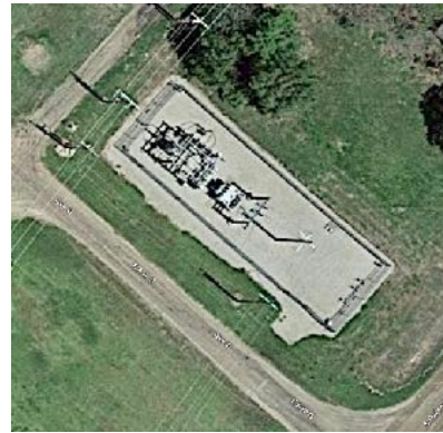
Nickerson Substation aerial
