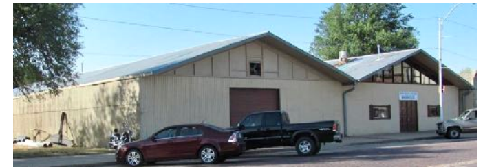
Southwestern Bell facility, Church, and USD 309 Warehouse
