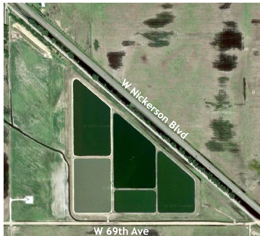
Aerial of Nickerson's Wastewater Treatment Facility
